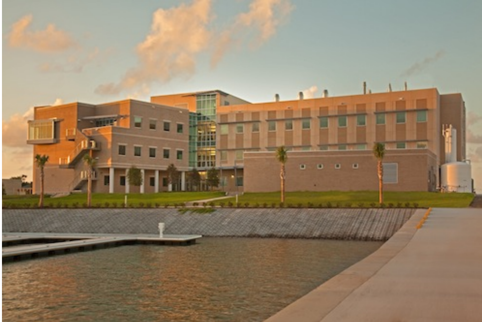
©WHR Architects, Inc./Carlo Macaione, photographer
